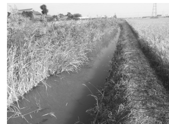
写真-2 多段（植生）護岸 Pic-2 Revetment covered with vegetation
